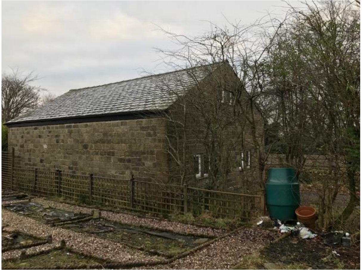
Garden - overlooked by skylights, enlarged windows and large glazing in lounge extension.
